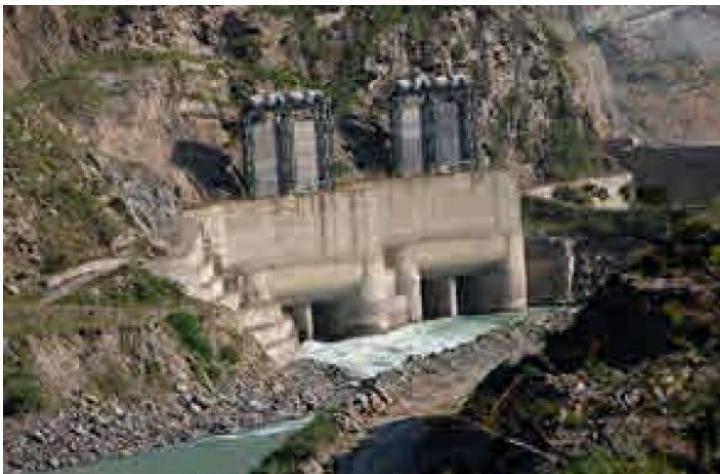
Top: Diversion tunnel for the Punatsangchhu Hydropower Project-I, Wangduephodrang.
