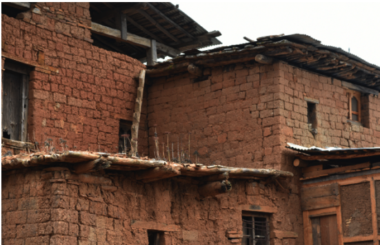
Figure 11. Houses constructed with mud bricks (Source: Authors)
