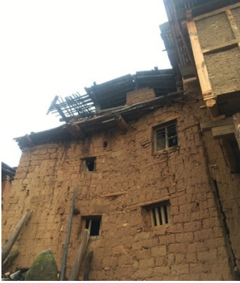
Figure 28. Mud Bricks as load bearing wall in Rinchengang (Source: Author)
