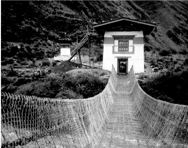
Fig. 33: The newly erected Tamchog Chakzam (2005) across the Paro Chhu.
