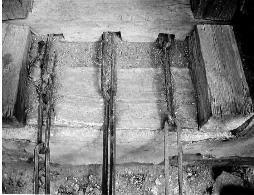
Fig. 35: The anchorage of the Doksum Chakzam
